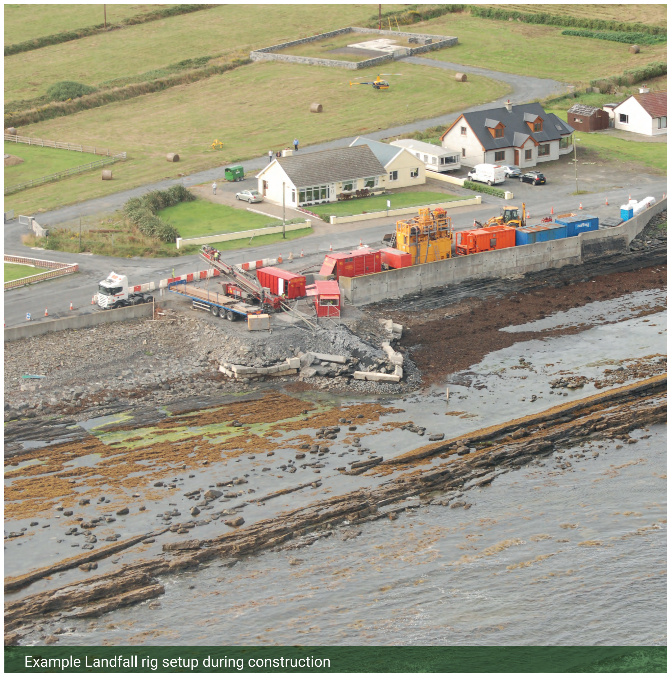
Example Landfall rig setup during construction
